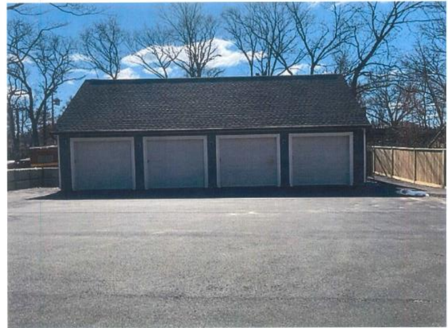
View of Garage located South/East
